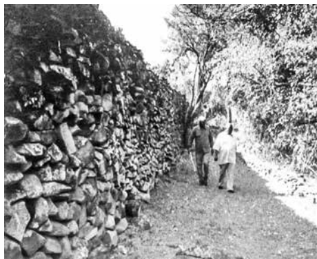
FIGURE 4 General view of main wall Source: Luby and Onjala 2012
