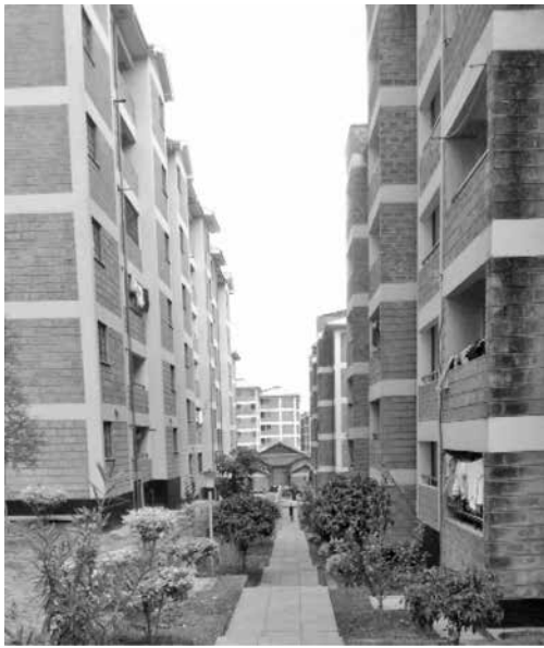
FIGURE 5 KENSUP housing flats Source: Author 2016
