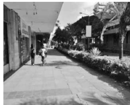
FIGURE 20 National Housing Corporation paved double walkway separated by vegetation Source: Authors 2017
