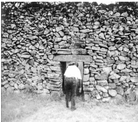
FIGURE 3 Walls and gate entry to enclosure Source: Luby and Onjala 2012
