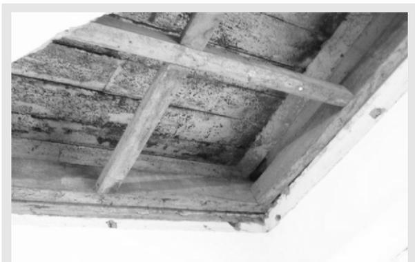
**Fig. 7: Damaged Kitchen Ceiling Building Interior**
